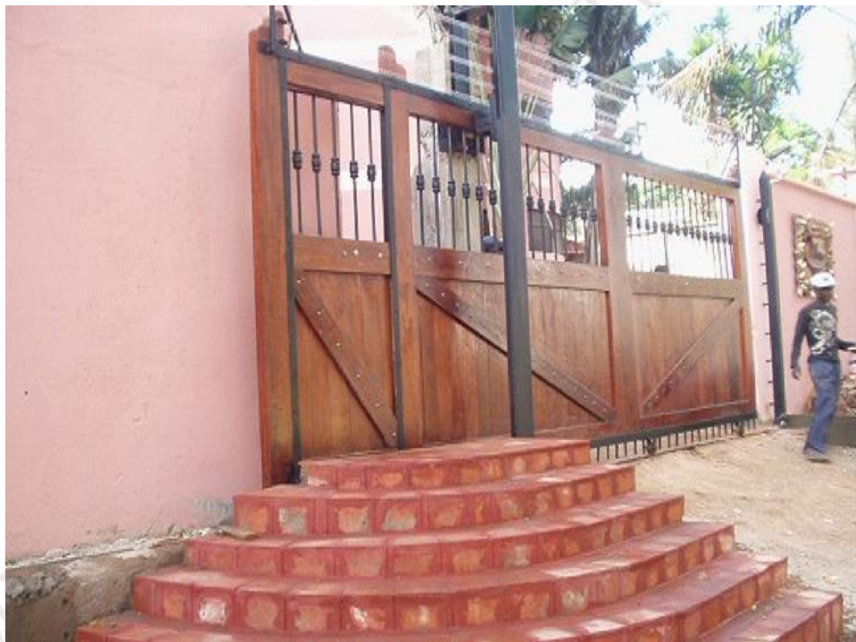
6m long wooden sliding gate at Wasini
