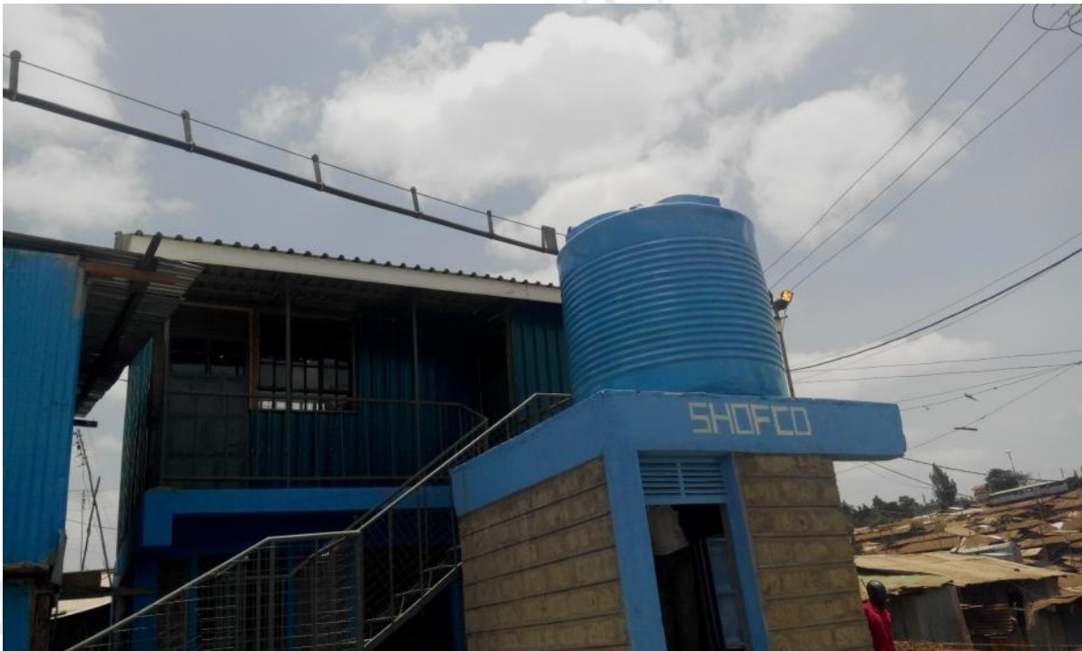
Aerial pipping for Shofco
