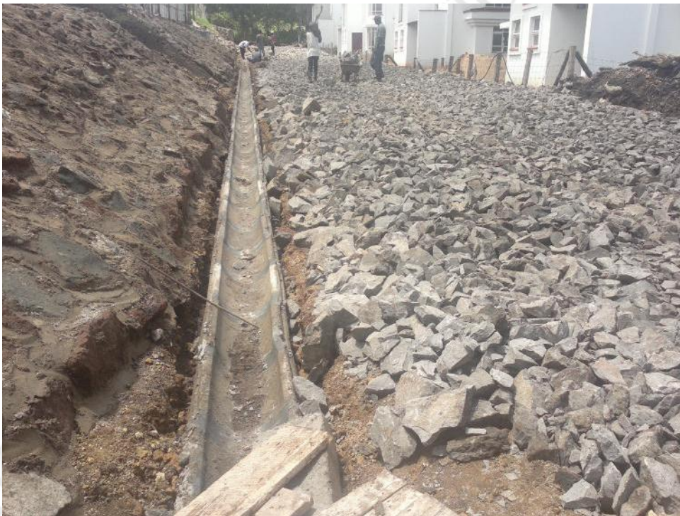
Photos of road construction in Kiserian
