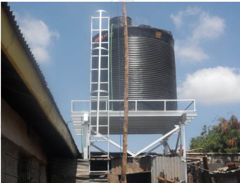
Water project for kisumu ndogo primary school in Gomongo
