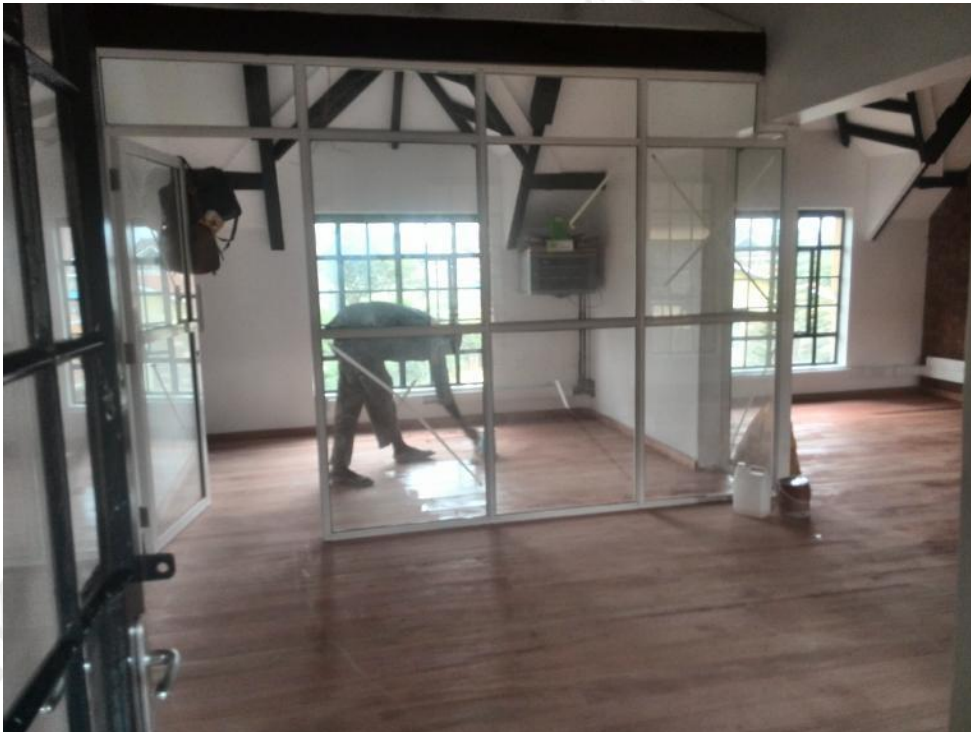
Aluminium partition and installation of timber floor board
