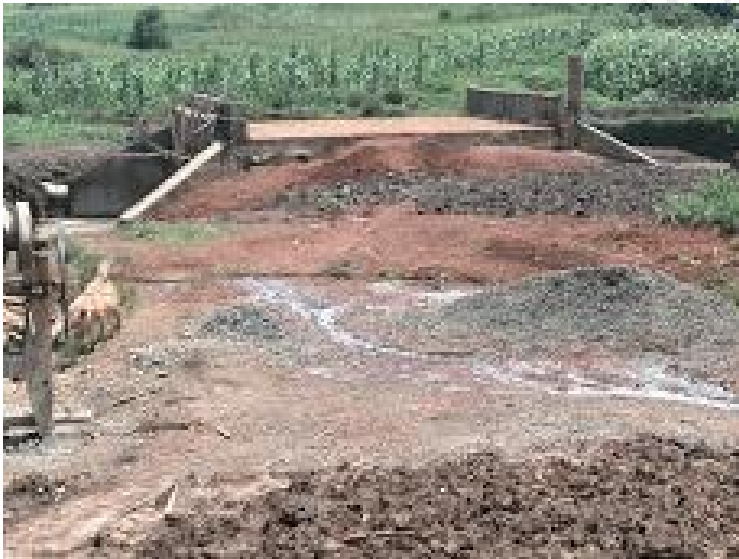
Box culverts for the Busia County project
