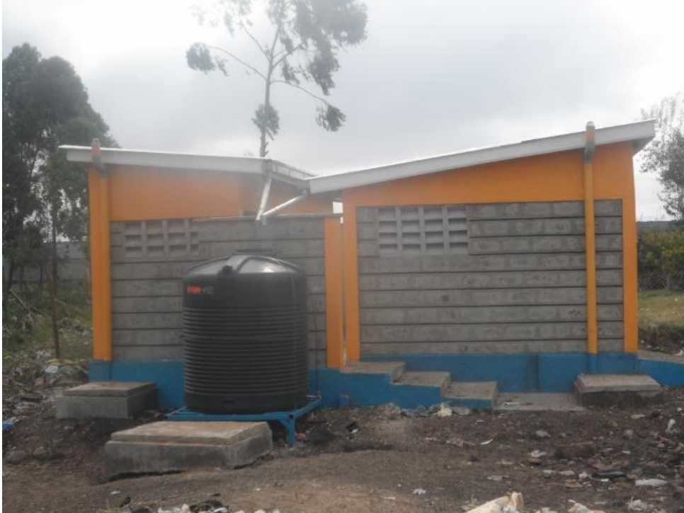
Toilet blocks for Menononite school in Mukuru
