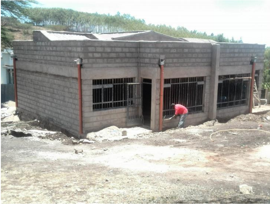
3 bedroom bungalow under construction
