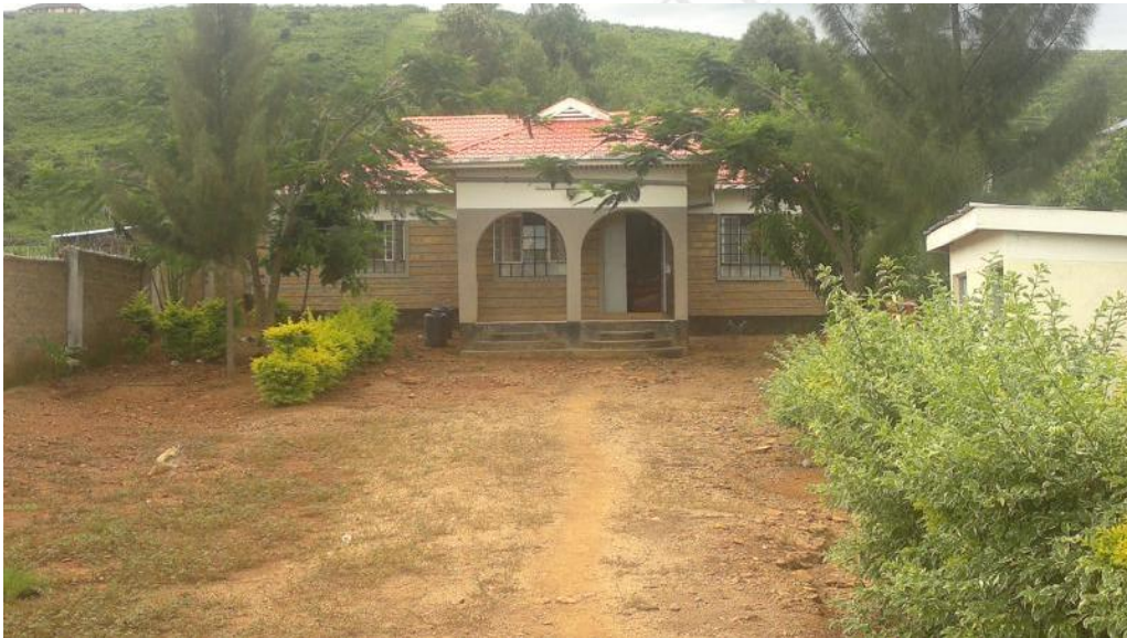
Residential House in Kisumu
